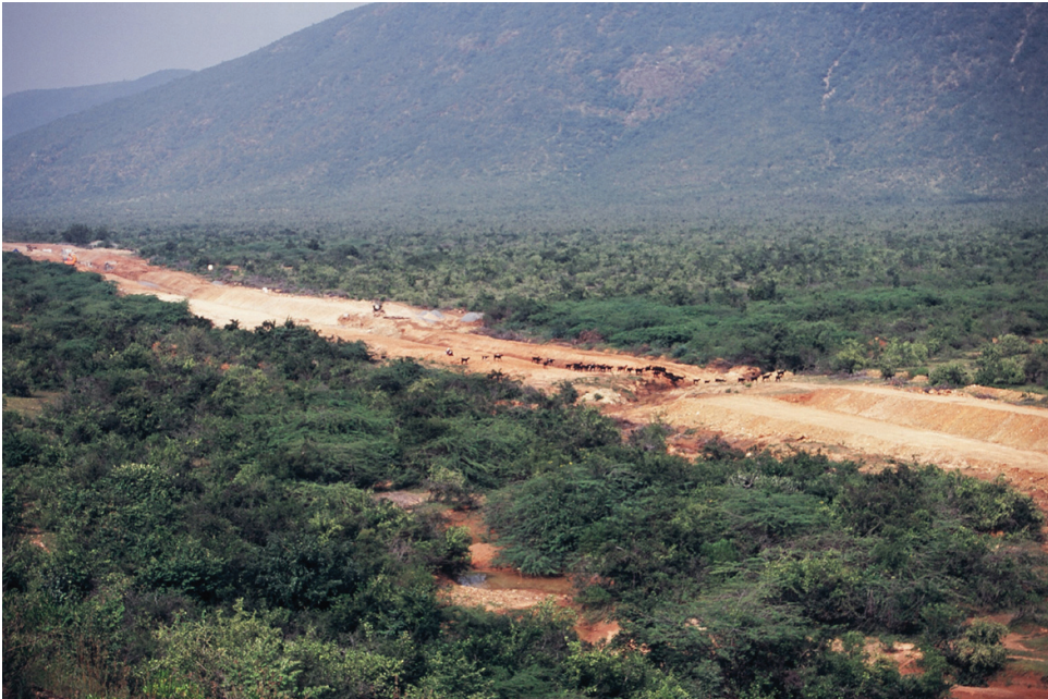
Several hectares of scrub jungle habitat around two protected areas, declared mainly for the Jerdon's Courser, was cleared for the construction of the Telugu-Ganga Canal
