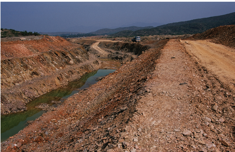
No permission was sought from the Andhra Pradesh Forest Department for clearing the scrub jungle habitat and for constructing the Telugu-Ganga Canal around the protected areas
